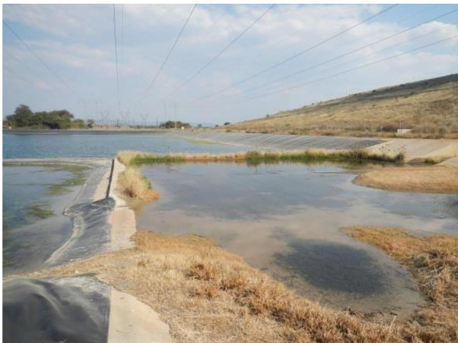
**Photo 15.2: Site Alternative 1 - Lined PCD (Sample Point MA SW 3&4)**
