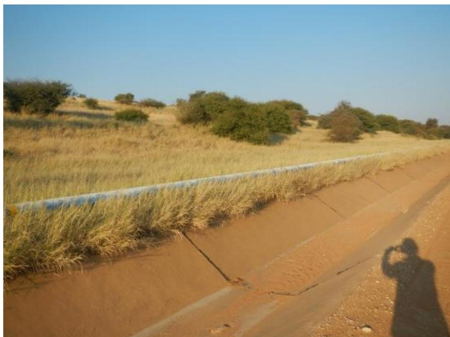
**Photo 15.4: Site Alternative 1 - Storm water trench next to rehabilitated Matimba Ash disposal site**
